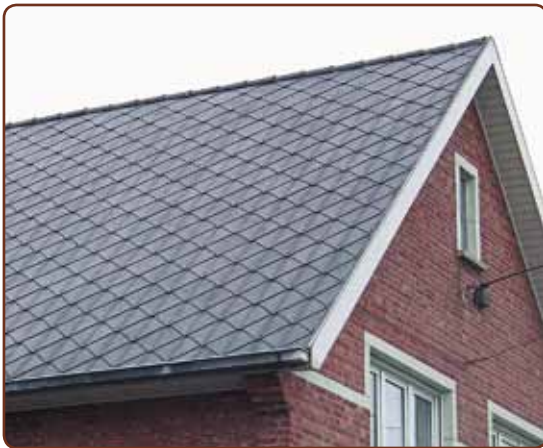
Dakleien in asbestcement
